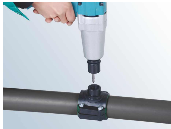
3. Drill a hole in the pipe wall, be carefull not to damage the thread and the O-
