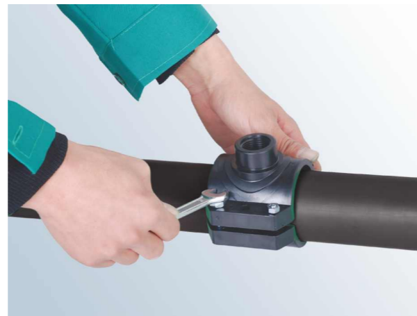
2. Position the bottom part of the saddle on the chosen point and couple the upper part, then insert the screws from below and tighten the nuts one by one.
